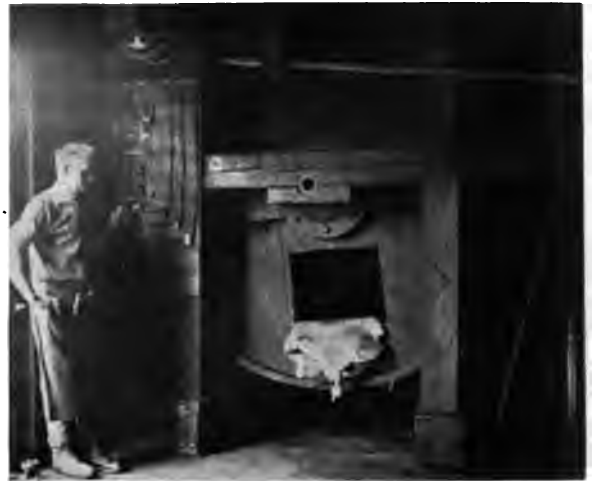
Fig. 2. Tanning Mill, driven by Individual Motor.
